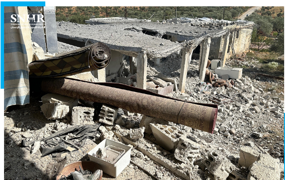
👁 Destruction and damage in Jafatlek Haj Hammoud village in western rural Idlib, following an airstrike by fixed-wing warplanes believed to be Russian - October 6, 2023 © SNHR
