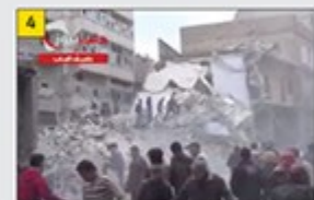
Second video recorded at the impact site of the first barrel bomb likely minutes after the explosion, matched with building damages in satellite imagery. http://www.youtube.com/watch?v=D r898oXkjsw
