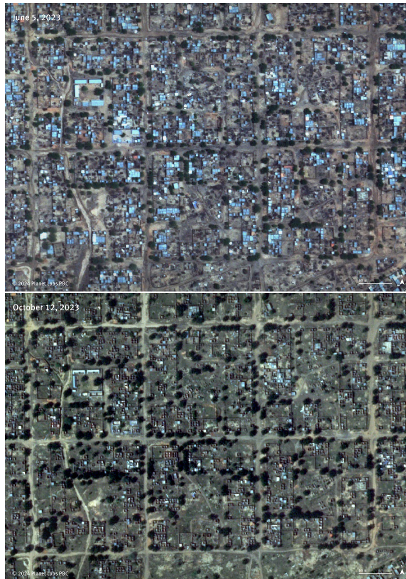
Caption: Satellite image comparison between June 5 and October 12, 2023, shows that rooftops on most of the buildings have been removed in an area illustrative of the destruction in the western part of al-Jabal neighborhood. Image © Planet Labs PBC.
