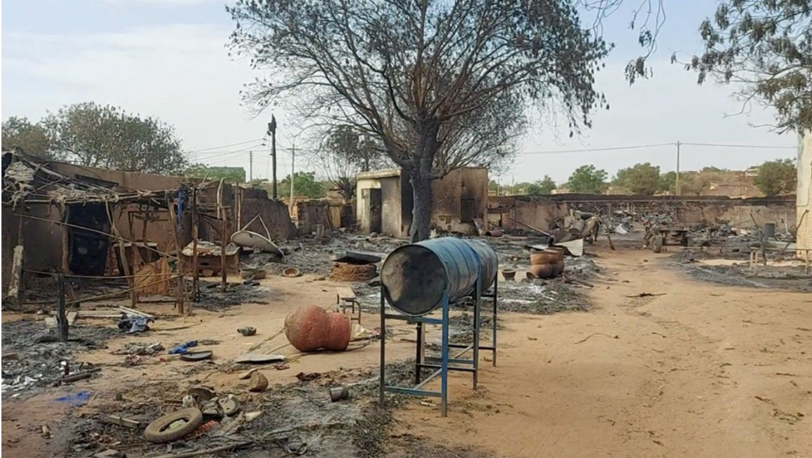
Incendiary damage to the Dar Massalit school, an IDP gathering site in El Geneina. © May 1, 2023, Roots for Human Rights and Monitoring Violations
