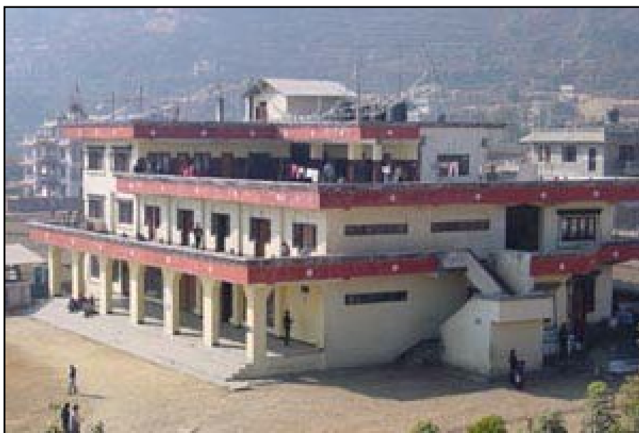
Figure 1: The Reception Centre in Kathmandu 7
