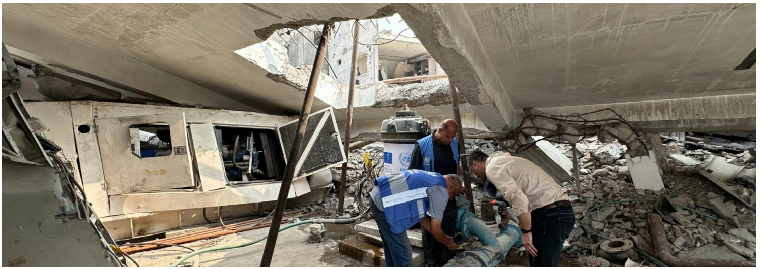
UNRWA teams repairing water infrastructure in Gaza. Photo: © November 2025 UNRWA
