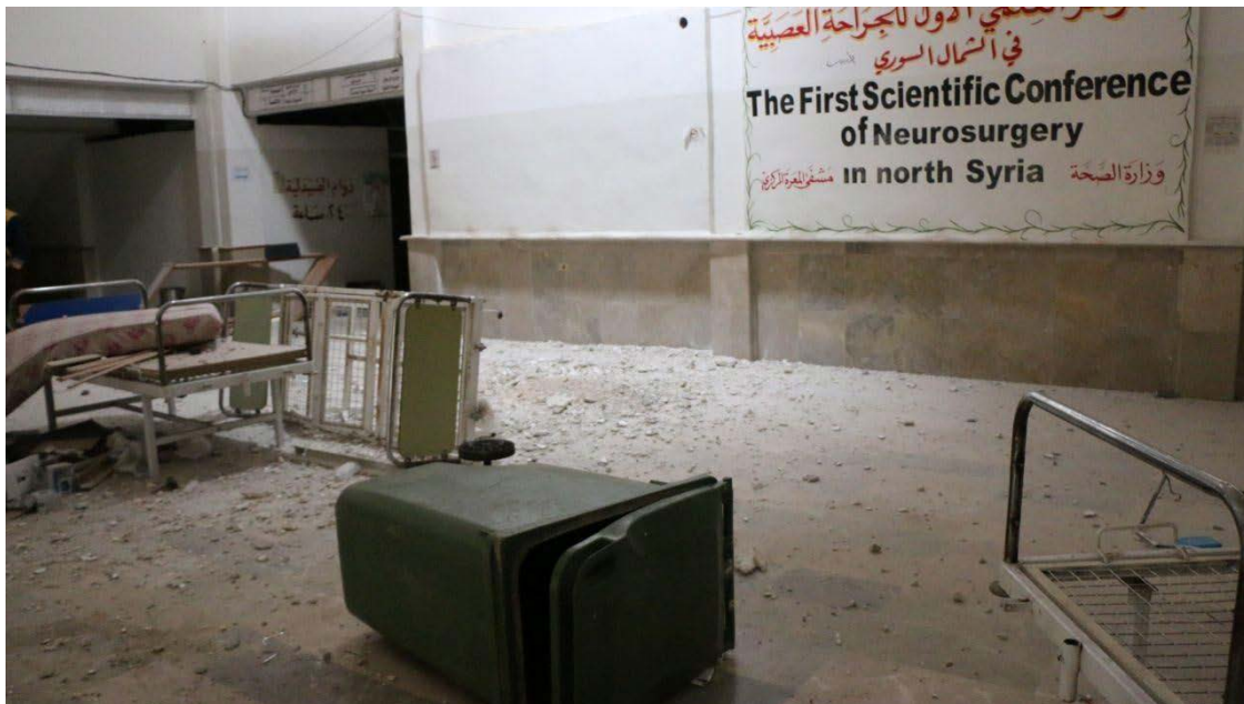
Early on January 8, 2020, munitions hit the roof, water tanks and yard of Maarat al-Nu`man National Hospital, the only functioning health care facility at that time. After the attack, the hospital stopped functioning. © 2020 Syrian Network for Human Rights
