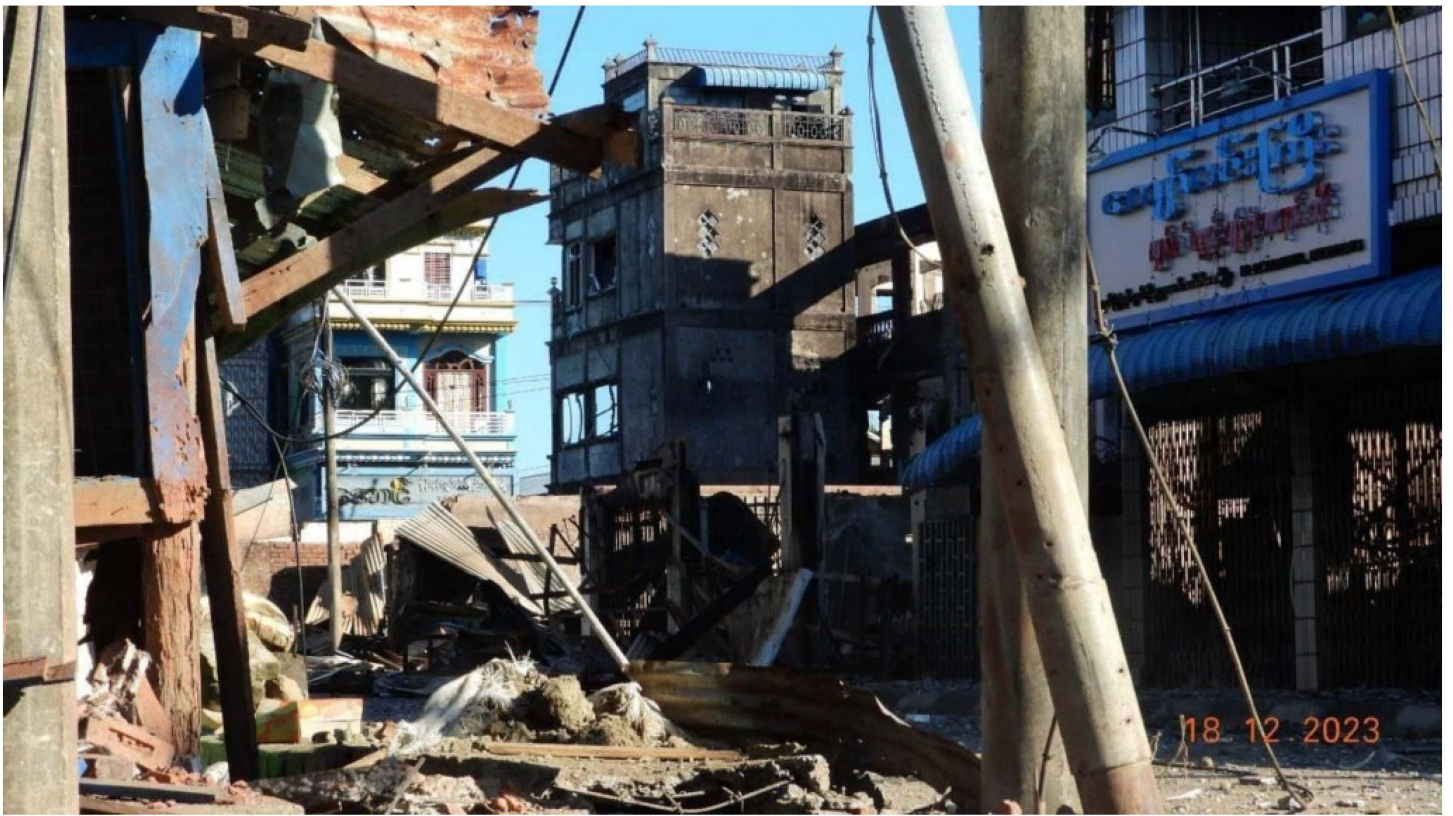
Damaged buildings in Pauktaw, Rakhine State, after weeks of fighting, 18 December 2023. © Private
