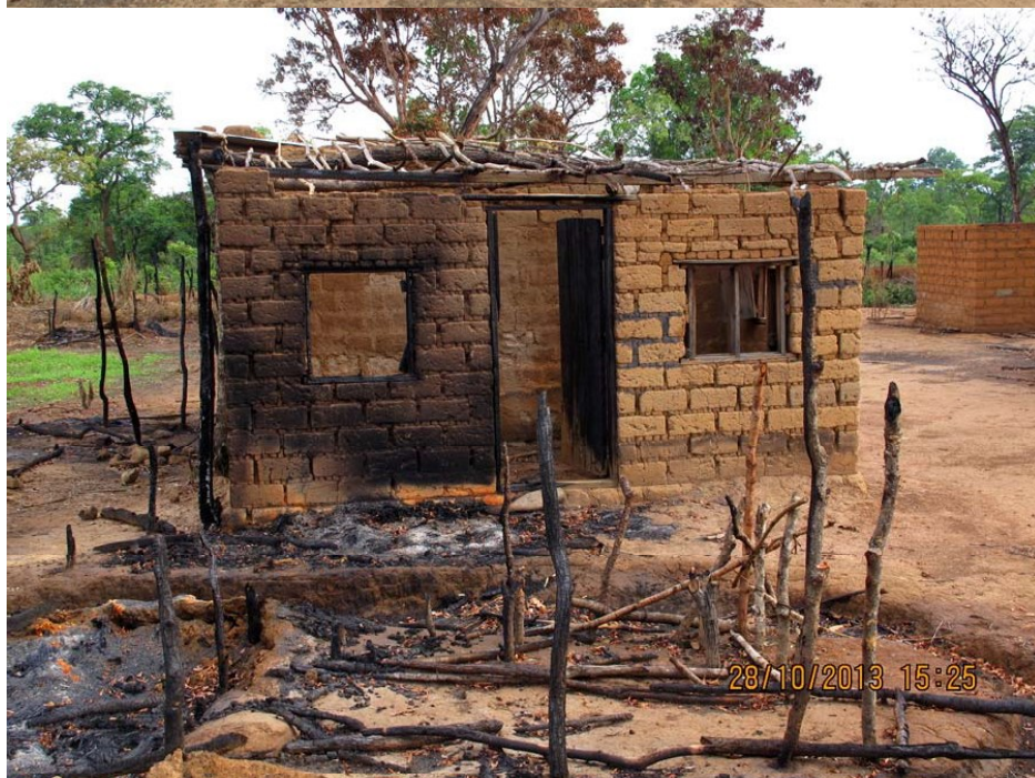
Burned structures in Kabola village.
