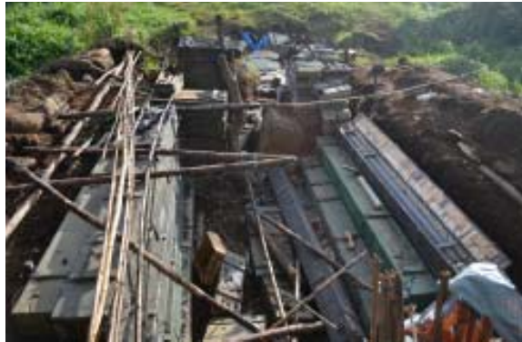
Location 1: storage of cannon shells and ammunition
