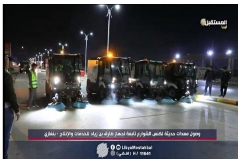
Figure 12.1 Road Maintenance in Benghazi
