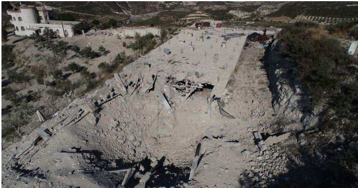
Destruction caused by a Russian aerial attack on a poultry farm in al-Shkheib village, Idlib - October 11, 2022
