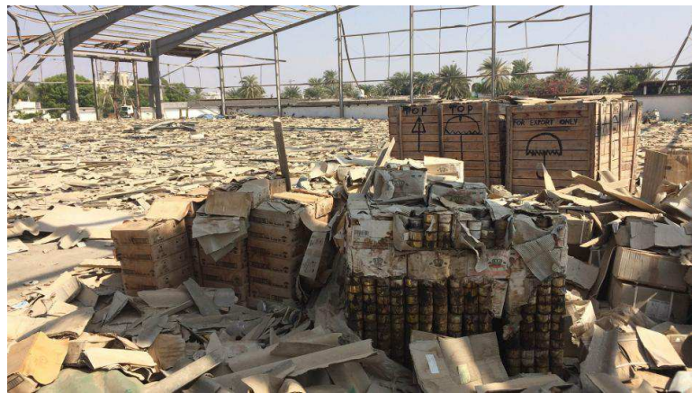
Imports sit destroyed in a damaged warehouse at the port in Hodeida city, Yemen.
