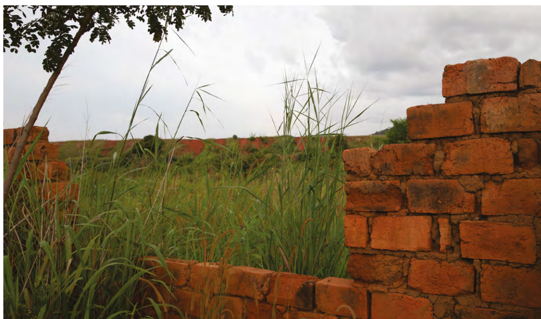
↑ House wall on an industrial mining concession, Kolwezi, February 2022 © Amnesty International (photographer: Richard Kent)
