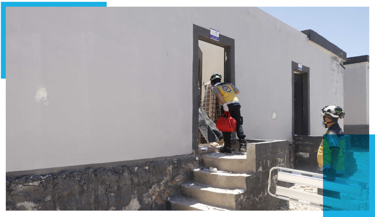
↑ 👁 Damage in a temporary IDP residential unit in the Ard al-Amal 'Land of Hope' village following an artillery attack by Syrian Democratic Forces (SDF) - May 8, 2024
