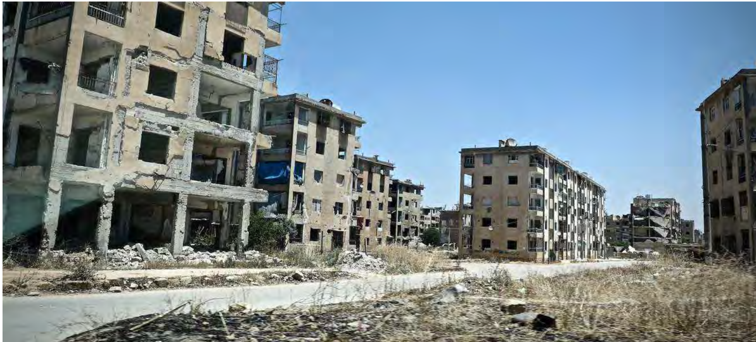
OCHA/Halldorsson | Destroyed buildings in eastern Aleppo city, Syria, where chemical weapons were allegedly used. (file photo)
