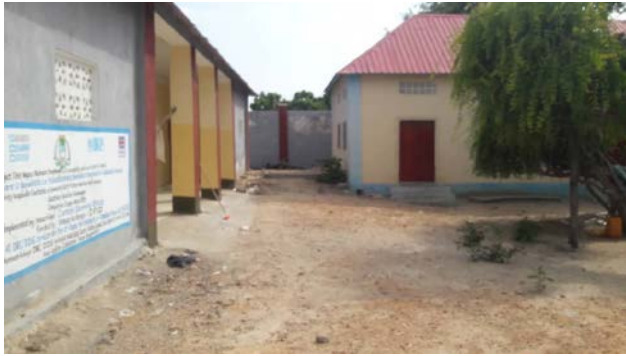
Photo: ADR facility in Kismayo, Jubaland
