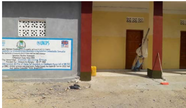
Photo: ADR facility in Kismayo, Jubaland
