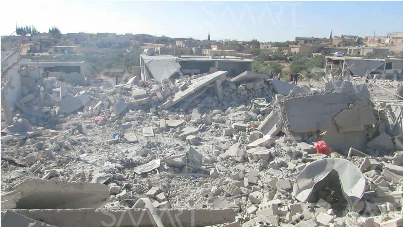
Massive destruction at Al-Tah town after being targeted by Syrian and Russian missiles
