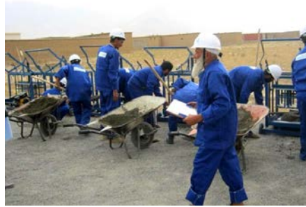
Training of returnees in concrete brick making 2011 © UNHCR
