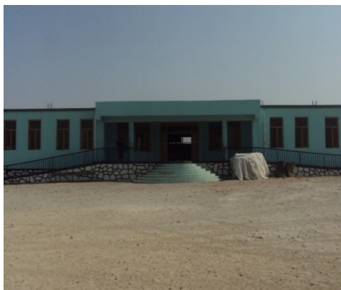
Front view of the school constructed by UNHCR@ AGHCO (UNHCR partner)
