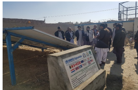
CBP program/UNHCR has Repaired Lavatory, dug bore well with solar system in Shahid Azimullah boys' high school/this picture is of the solar system installed for getting water through submersible from the dug bore well/ joint visit of UNHCR, DoRR, DoE and OHW/PARR-Loya Wala-PD# 09/Nomylai Aryan
