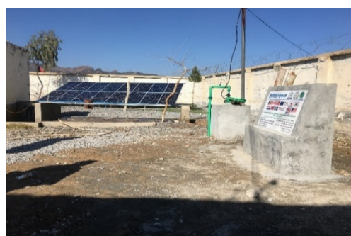
UNHCR dug bore well and provide Solar system to Abdul Shakur boys school to solve their water challenge/PARR-Mirwais Mina-PD#07/Iqbal Ferafhand-Liaison Officer
