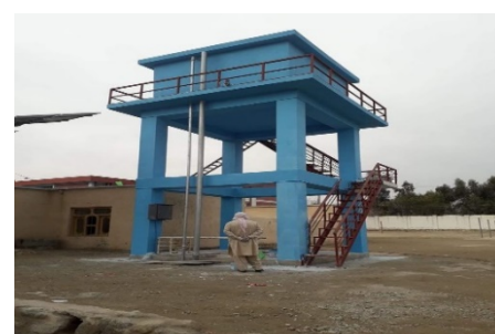
View of the recently constructed solar powered pipe scheme in Charbagh boys' school. © UNHCR partner/ Majeed
