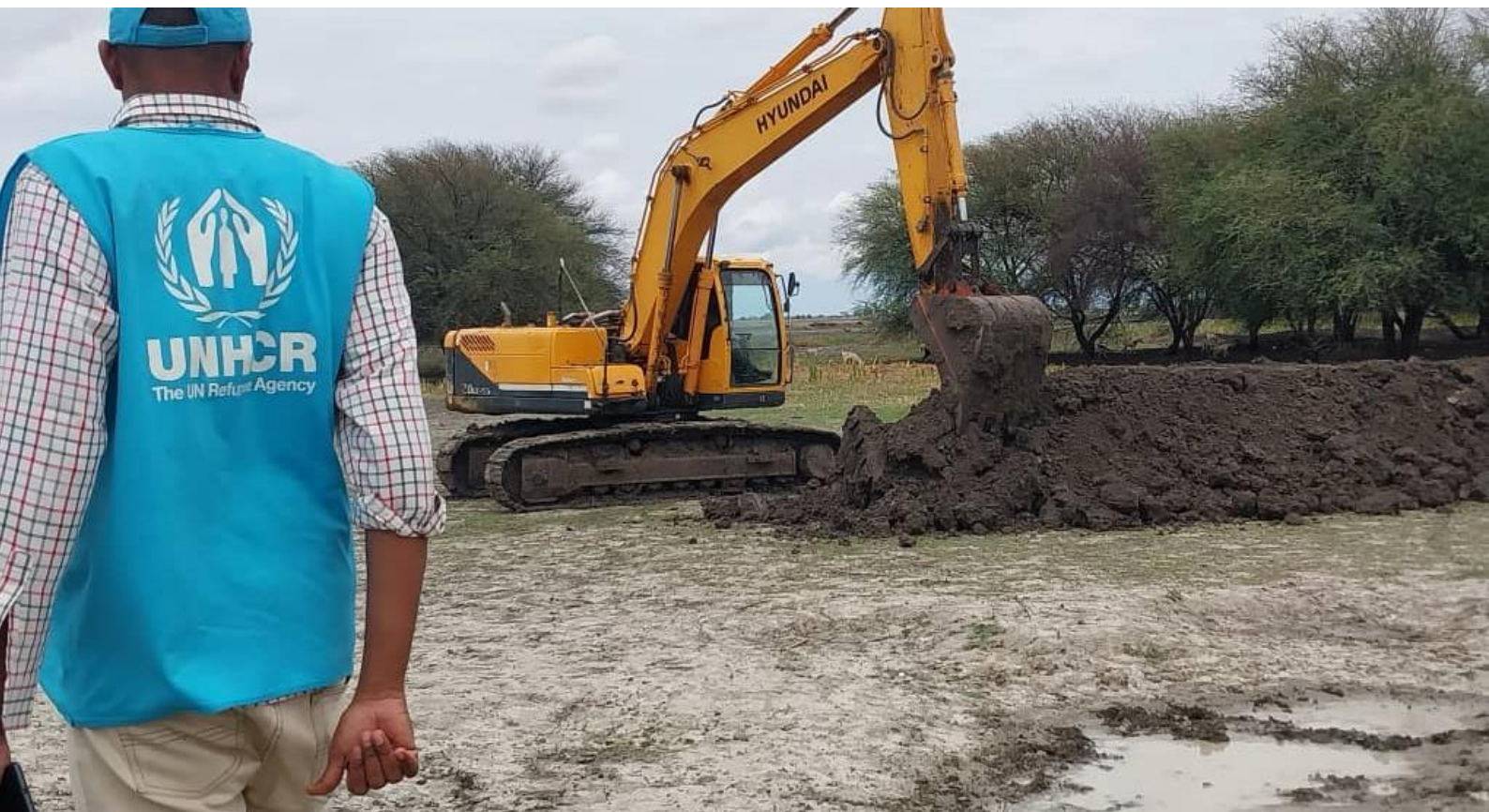
Ongoing flood mitigation work in various camps in White Nile State in anticipation of the rainy season. Photo: ADRA
