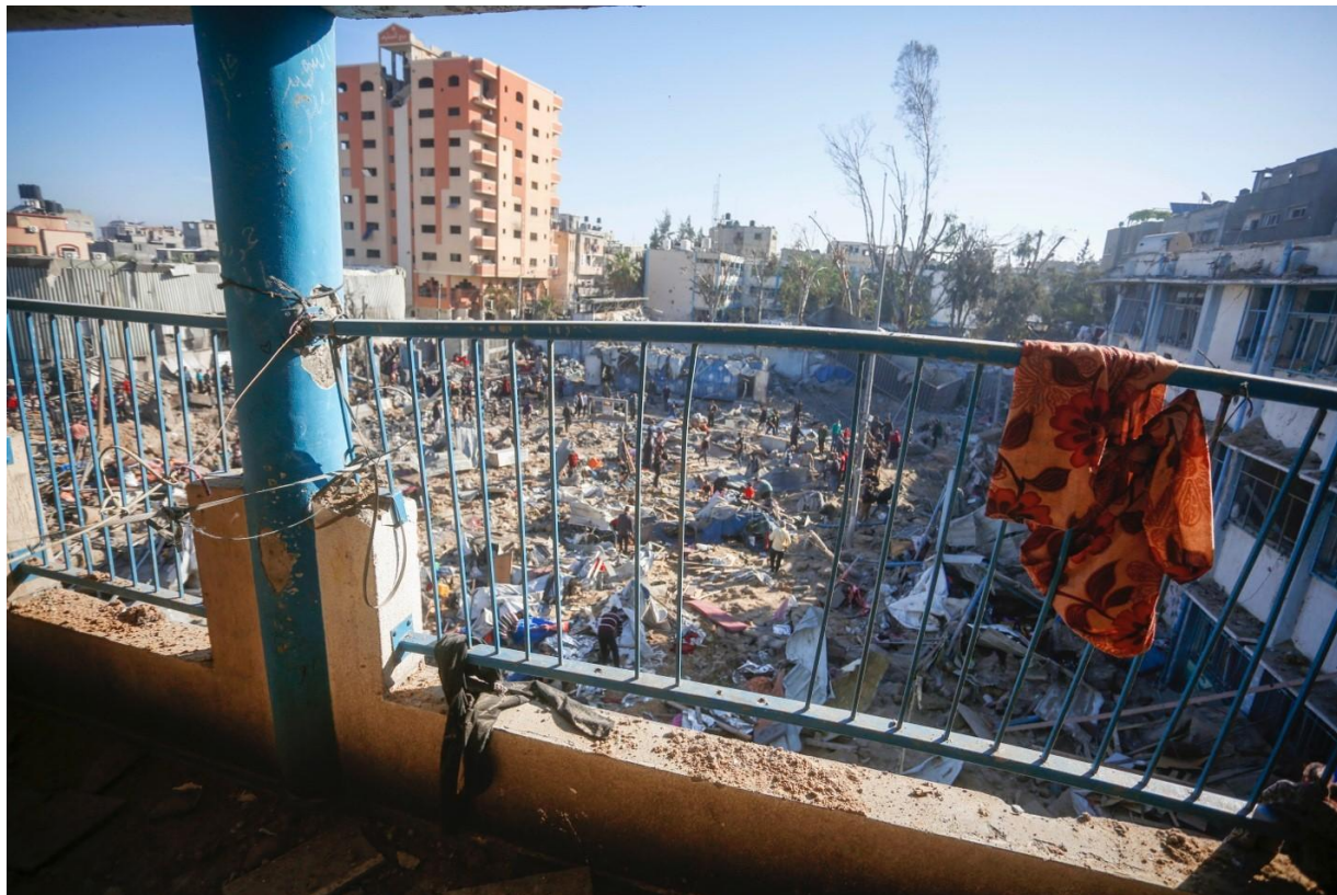
An UNRWA school-turned-shelter sustains severe damage after being hit twice by the Israeli Forces on 6 May 2025, Gaza middle areas, the Gaza Strip, May 2025. © 2025 UNRWA photo by Ashraf Amra
