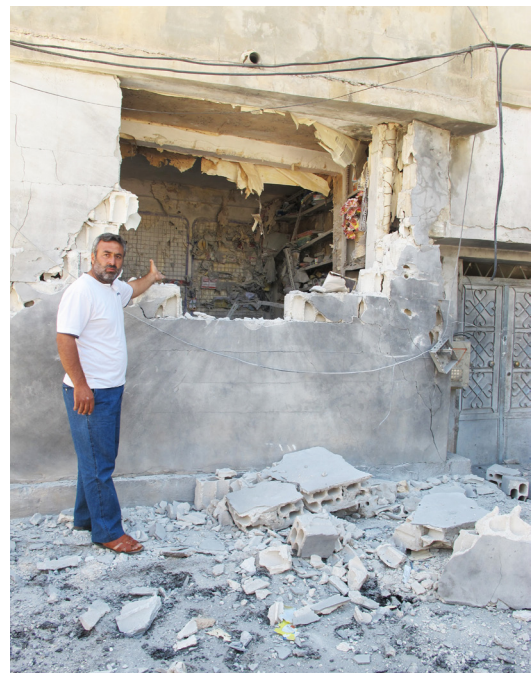
A resident of Homs, Syria, shows a building heavily damaged in the renewed rounds of shelling from early June 2012. (Photo: UN Photo/David Manyua)
