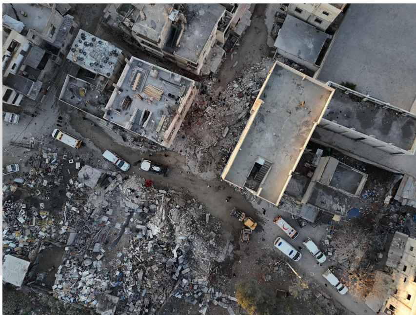
↑ 👁 A residential building destroyed in the aftermath of the explosion of a rocket from remnants of war inside the building in al-Raml neighborhood in Latakia city – March 15, 2025
