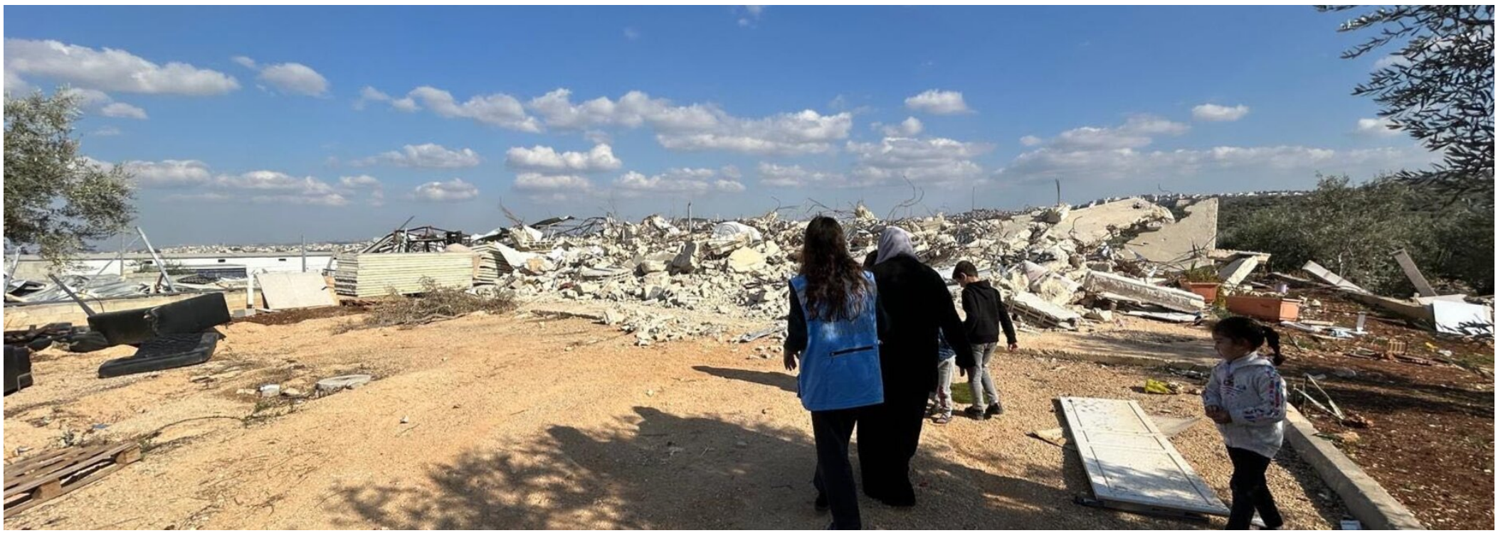
A Palestinian family from Deir Ballut, Salbit, shows an aid worker the three agricultural structures demolished by the Israeli Civil Administration, 17 December 2024. Photo by OCHA
