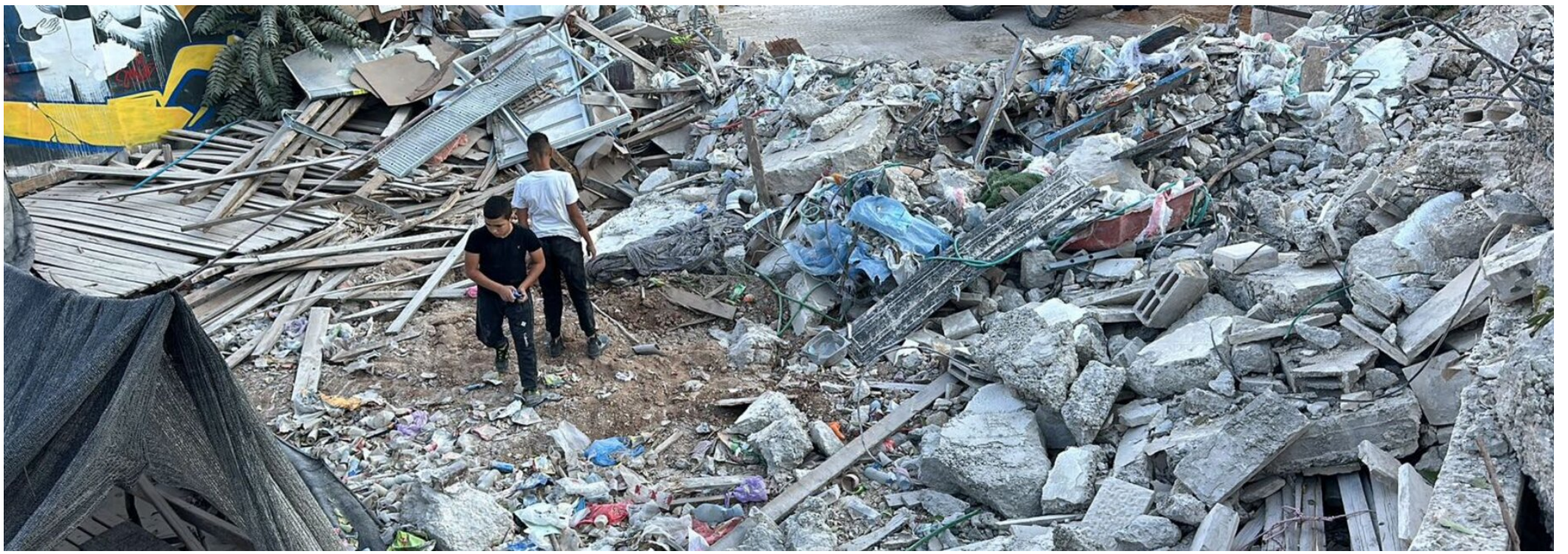
A demolished residential building in Al Bustan area of Silwan, East Jerusalem, hosting a community centre that served about 1,000 people. Photo courtesy of the community
