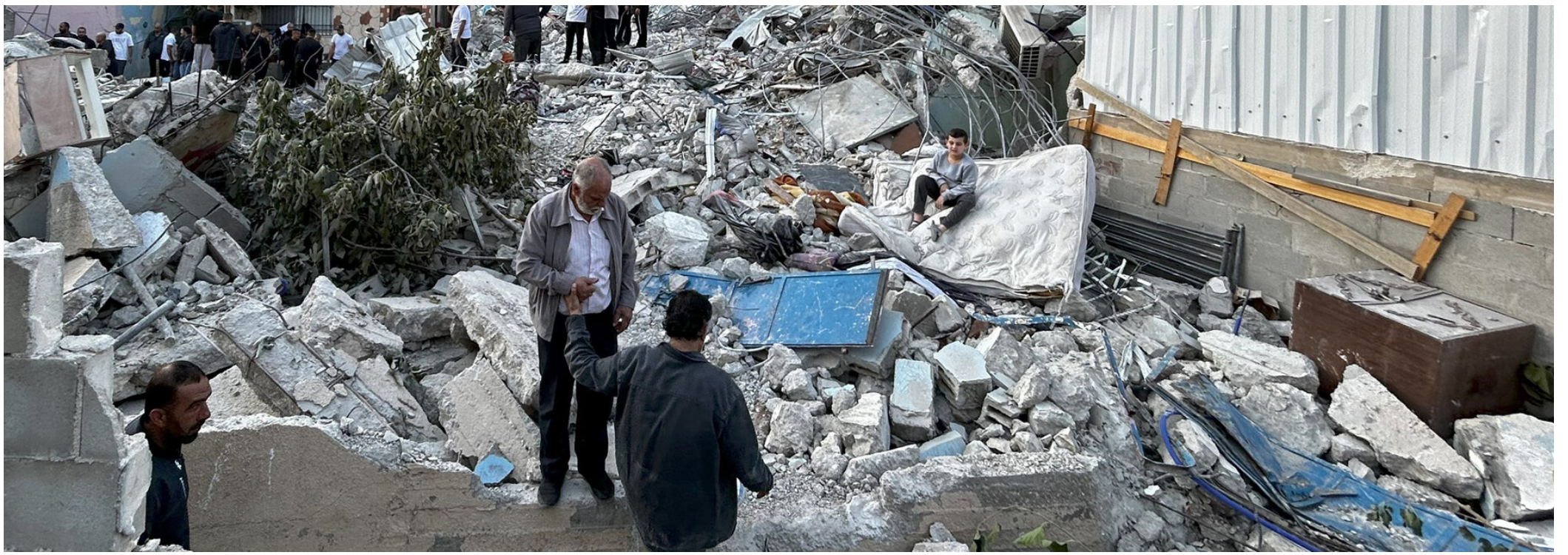
Al Bustan area of Silwan, East Jerusalem, where 42 Palestinians, mostly children, were displaced on Tuesday when Israeli authorities demolished nine homes. "We have nowhere else to go," said one resident. "We will sleep on top of the rubble." Photo by OCHA
