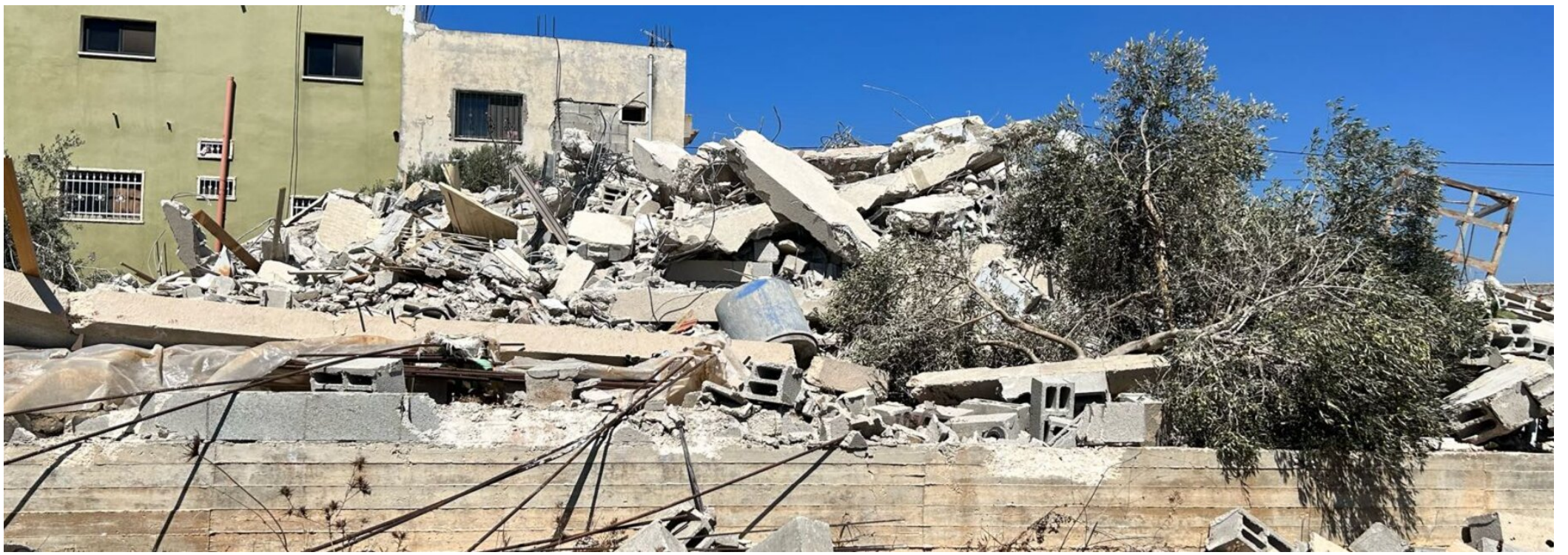
A two-storey home demolished by the Israeli authorities in Tura ash Sharqiya (Jenin) on 24 September, displacing a girl and her parents. Photo by OCHA
