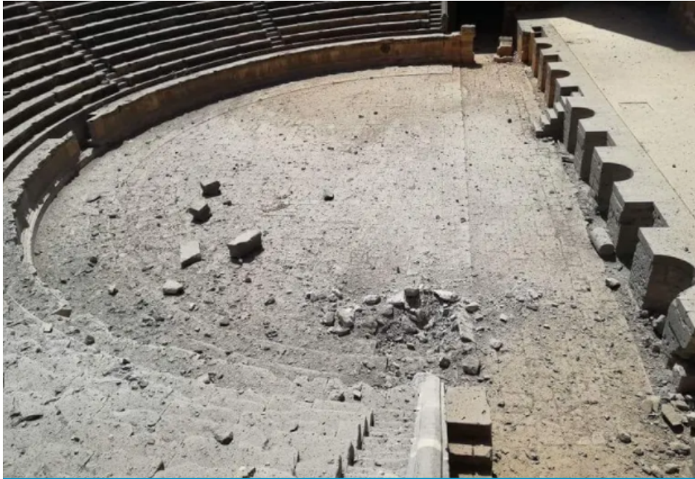
Destruction inflicted by the Syrian Regime attack on Roman Bosra Theatre in Bosra al Sham city, Daraa – July 1, 2018
