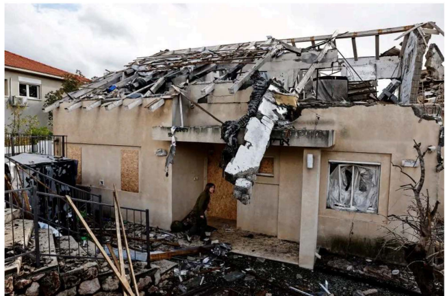
A destroyed structure in Metula, which became the site of heavy rocket barrages from Lebanon, amid cross-border hostilities between Hezbollah and Israel, November 18, 2024.
