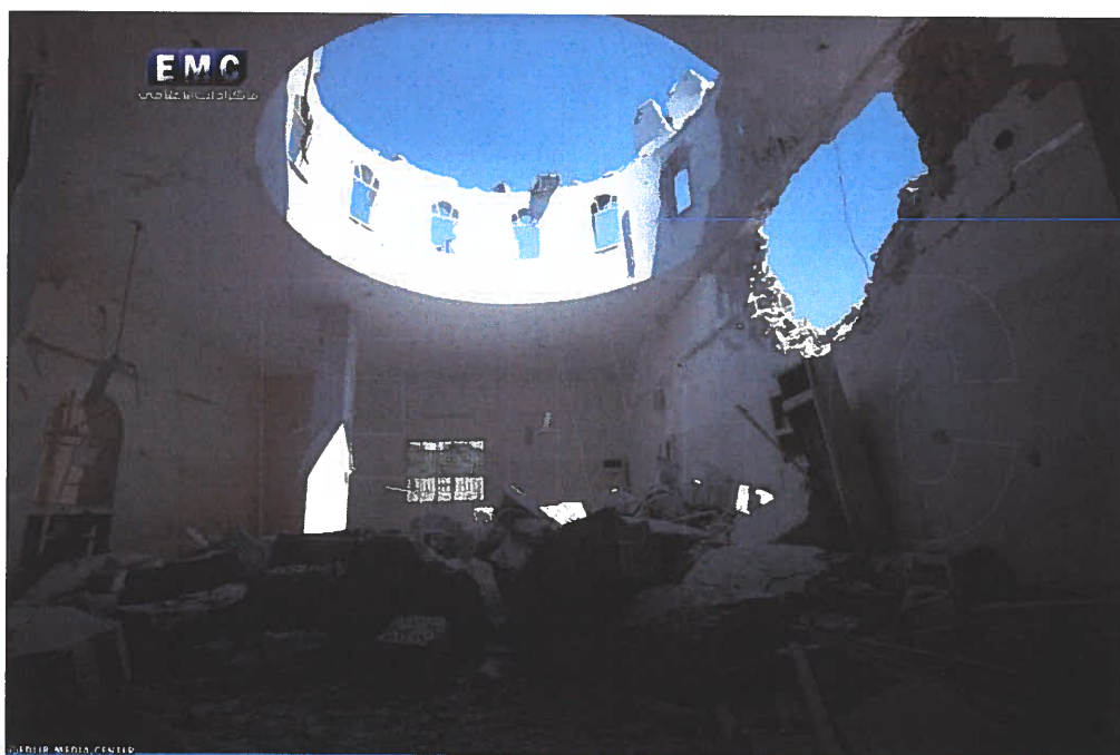
Destruction in Abu Bakr al Siddiq Mosque in a Syrian air attack on Khan al Sebel village, Idlib – May 28, 2019
