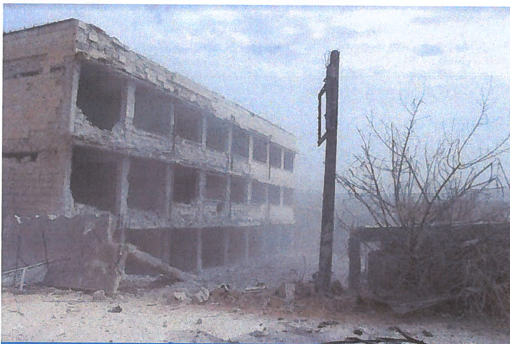
Destruction in Ruqayya Bint Malek High School in a Syrian air attack on Kafranbel, Idlib – May 22, 2019
