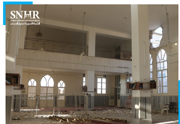
👁 Destruction to the Omar bin al-Khattab Mosque in Oulshalli village in Aleppo following a ground attack by the SDF - September 6, 2023 ©SNHR
