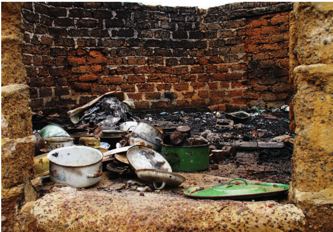
A burnt house in Ziléby village, which was attacked on March 13, 2013 by people who crossed over from Liberia. The attackers appeared to target people who were seen as associated with allegedly illegal land sales that stripped refugees of their land. April 26, 2013. © 2013 Tamasin Ford
