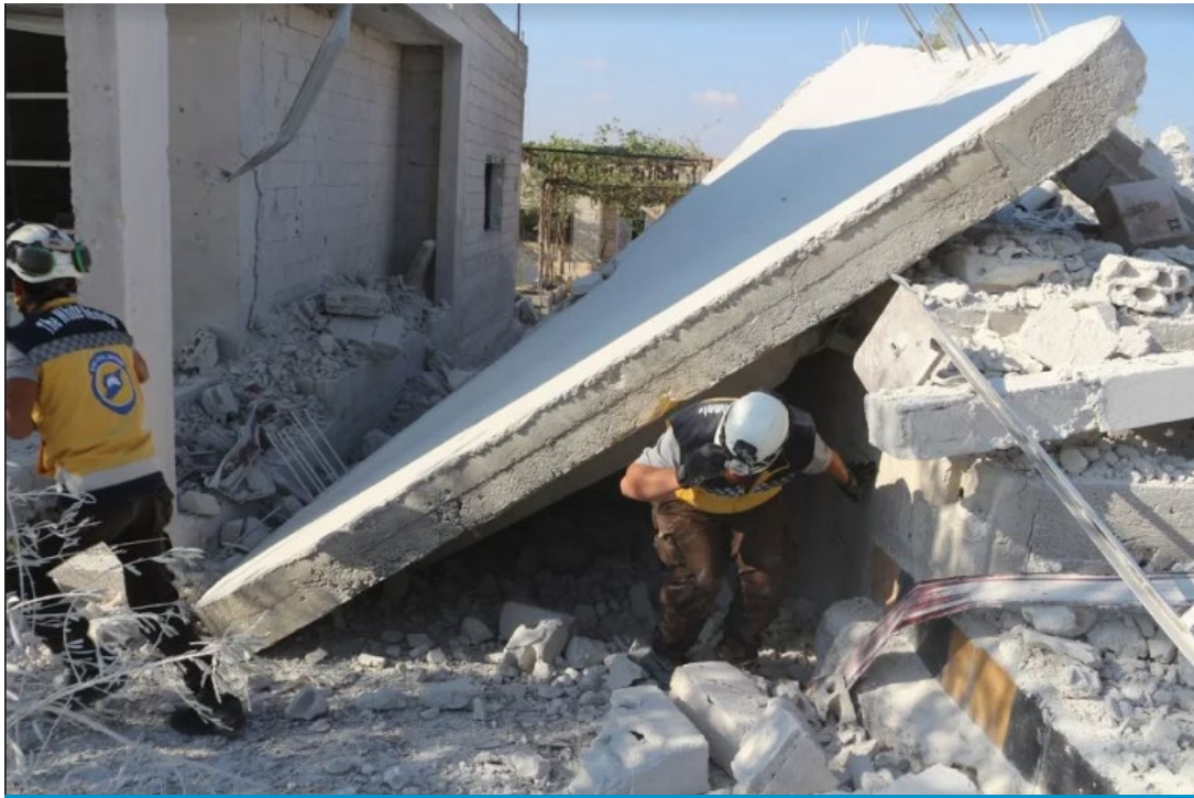
Destruction caused by an air raid by the Syrian regime on the Civil Defense Center in Sfuhun village, Idlib - September 12, 2019
