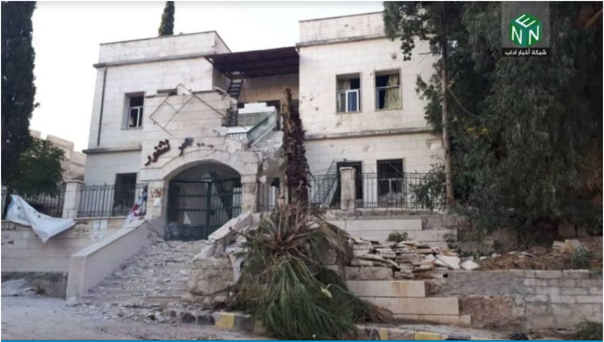
Destruction to the Dispensary in Jisr al Shoghour city, Idlib, caused by Syrian regime's ground attack – November 4, 2019
