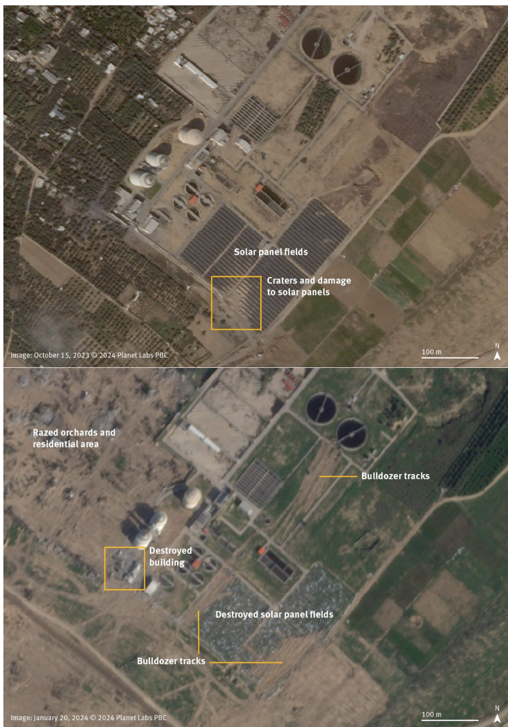
Satellite imagery comparison between October 15, 2023 and January 20, 2024 shows the progressive destruction of the Central Gaza wastewater treatment plant. Solar panels were first damaged in early October 2023 before being destroyed in November. As of January 20, 2024, one of the main buildings was completely destroyed and several areas of the plant appear to have been razed by bulldozers. Images © 2024 Planet Labs PBC. Graphics and analysis © Human Rights Watch.
