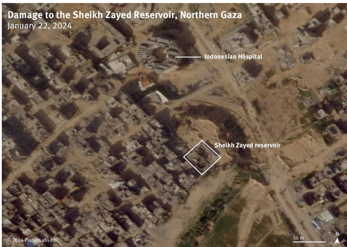
Satellite imagery from January 22, 2024 shows the damage to the Sheikh Zayed reservoir, located in northern Gaza, 150 meters south of the Indonesian Hospital. Both main buildings of the reservoir show large damage impacts on their rooftops. Image © 2024 Planet Labs PBC
