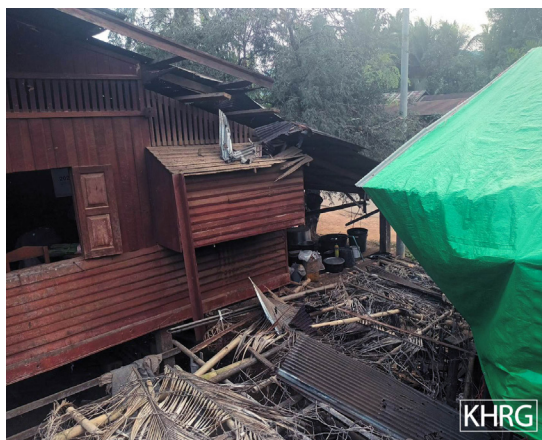
This photo was taken on March 24th 2022 in Htee Moo Hta village, Noh Hpoh village tract, Kaw T'Ree Township, Dooplaya District. It shows a house that was damaged by indiscriminate shelling undertaken the same day by SAC LIB #355 during an armed clash. A 17-year-old girl was killed and three other villagers were wounded in the attack. [Photo: KHRG]
