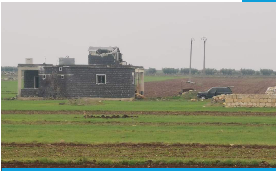
↑ 👁 Damage to a house caused by a ground attack by Turkish forces on Abin village in Aleppo - February 12, 2024
