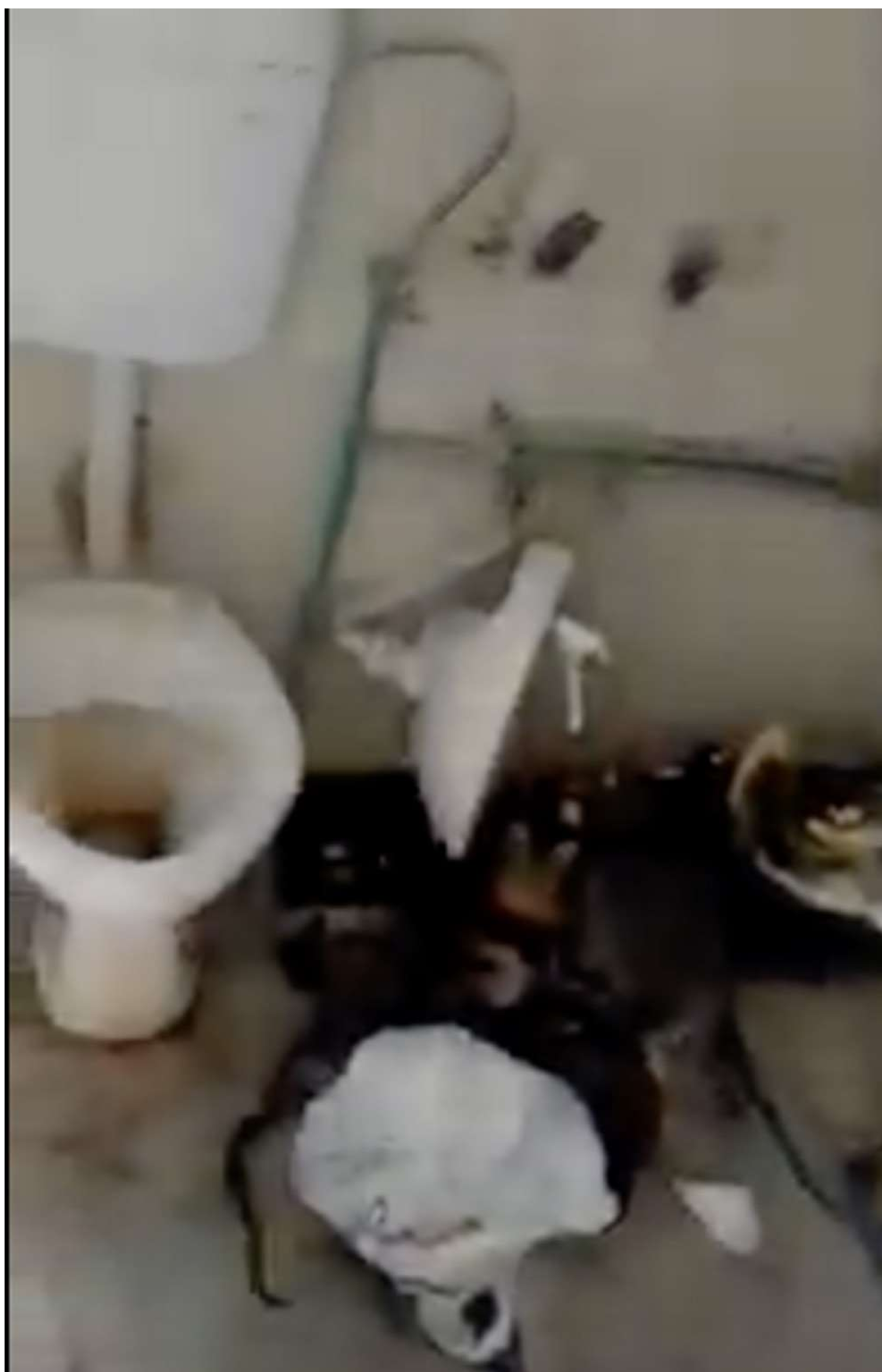
Toilets in Amygdaleza PRDC
