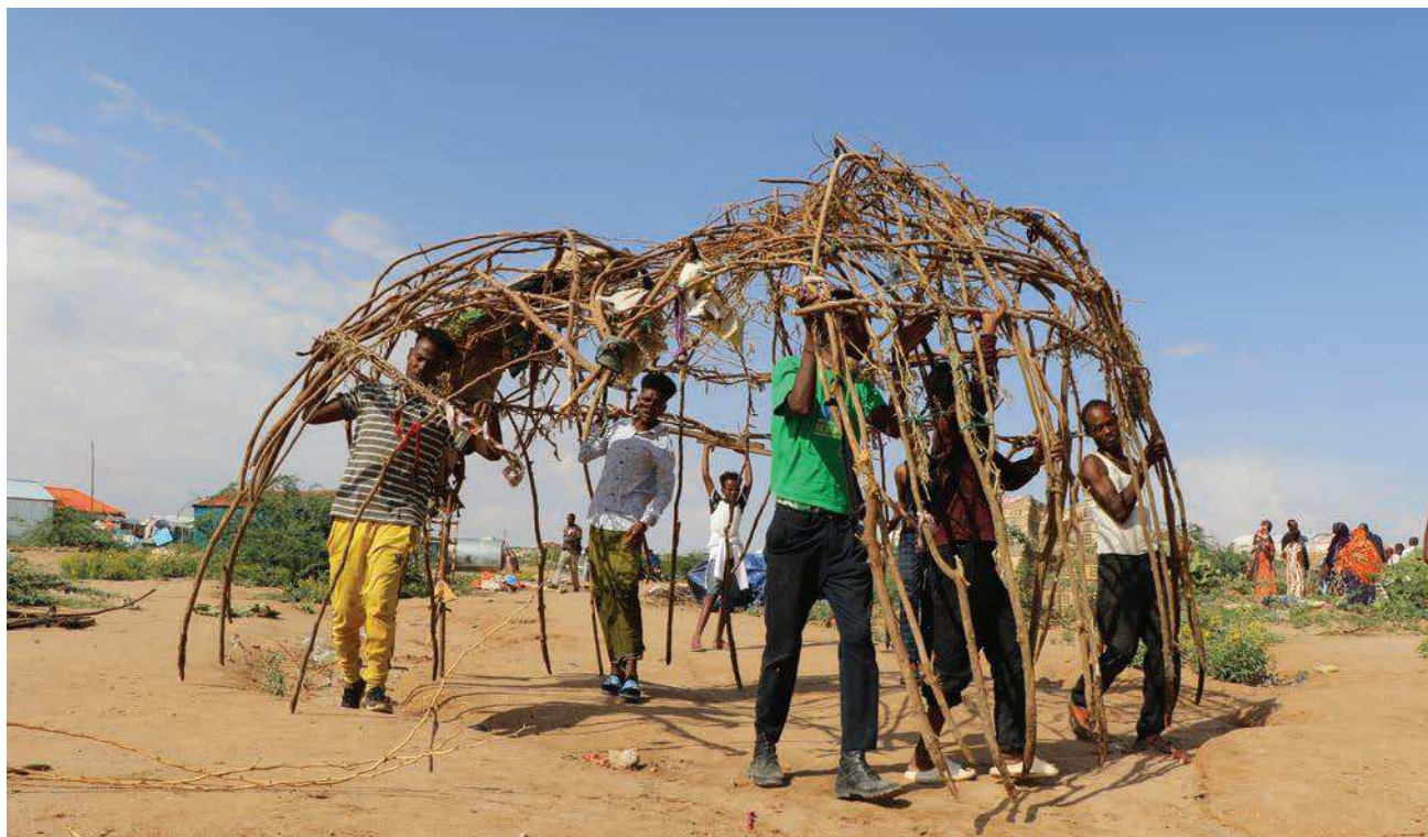
Group of men constructing a shelter structure
