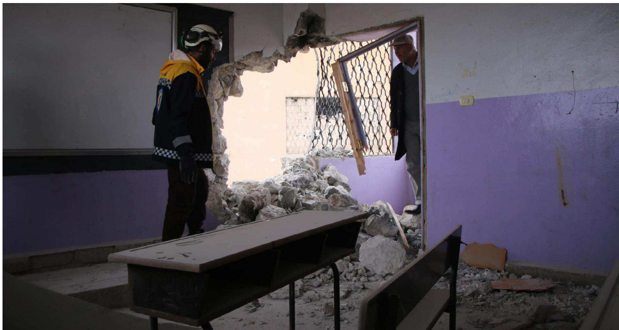
Destruction in the aftermath of a land attack by Syrian regime forces on Ma'ar Ballit Halqa Oula School in Ma'ar Ballit village, Idlib - November 4, 2022
