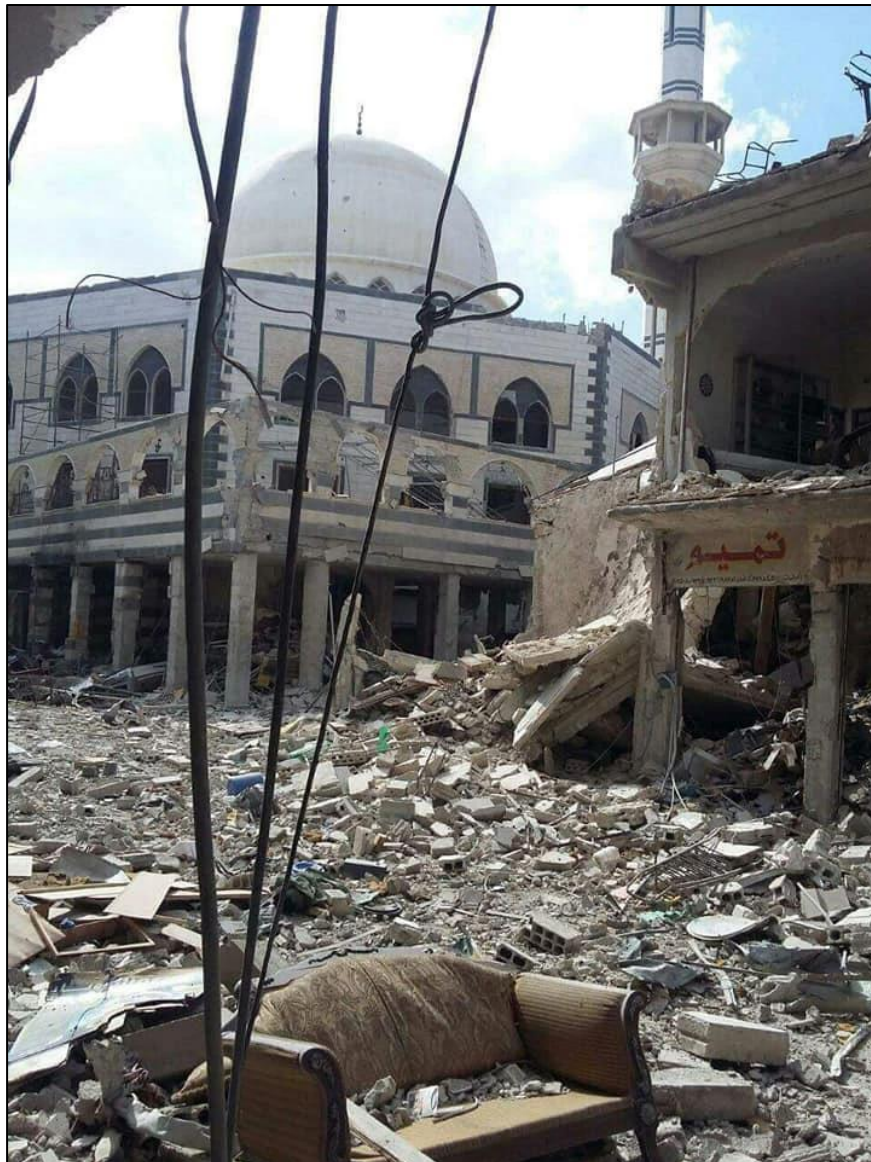
Damage left by shelling on Yarmouk Camp in Damascus (photo: 22/4/2018)
