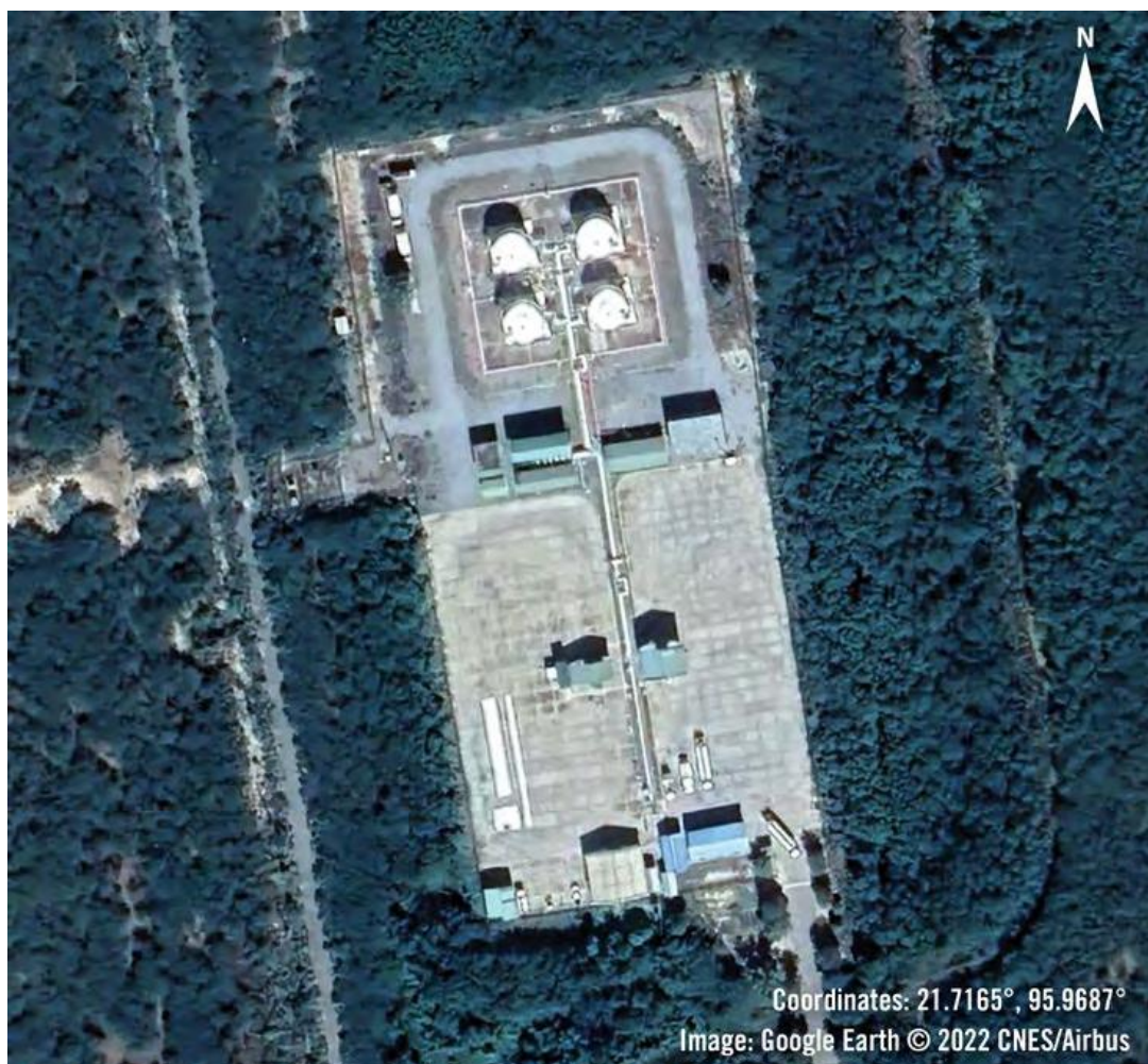
NEPAS storage facility at Mandalay airport.
