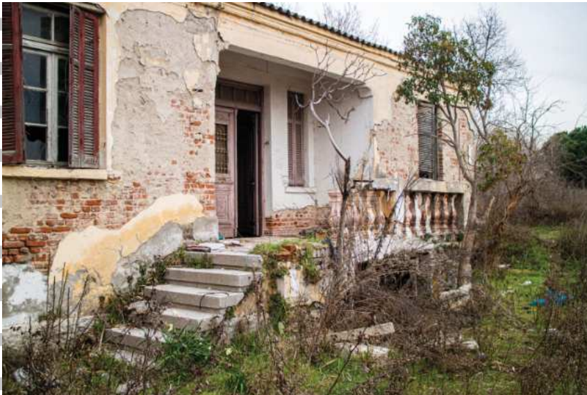
Abandoned building, Thessaloniki and surroundings Benj Herren 2021
