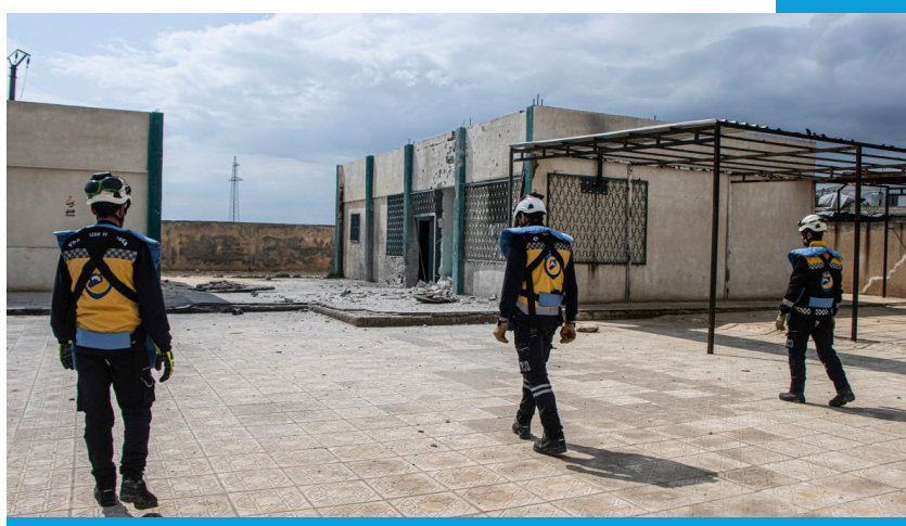
↑👁 Destruction caused by a ground regime attack Murshed Mohammad Ayyan Elementary School in Katyan village in Idlib - March 19, 2024
