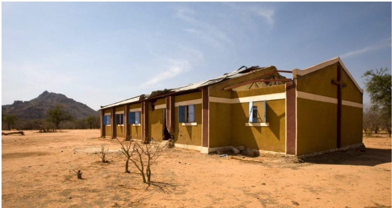
The Kurada Sudanese Church of Christ building, destroyed by a jet fighter from the Sudanese government in November 2014, Tojor village, Dalami county, South Kordofan, Sudan. January 2015. Photo: Giovanni Diffidenti
